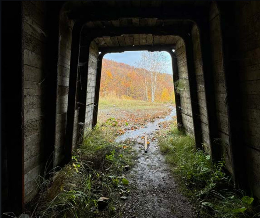
Looking out from the adit
